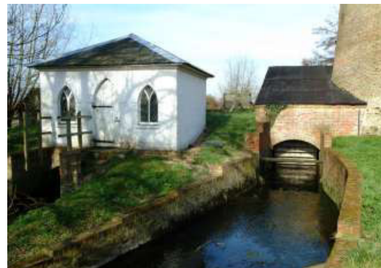
The pumphouse, March 2003
