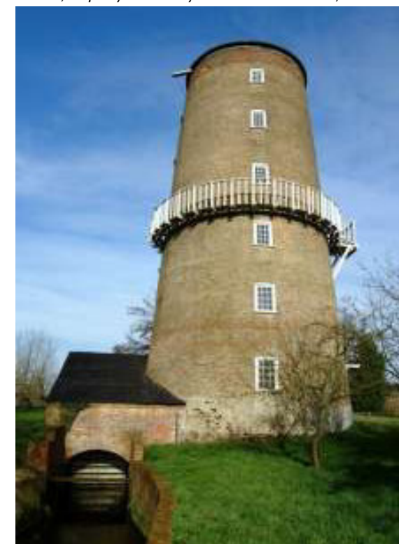
The Mill, as partly restored by Norfolk Windmills Trust, 2003
