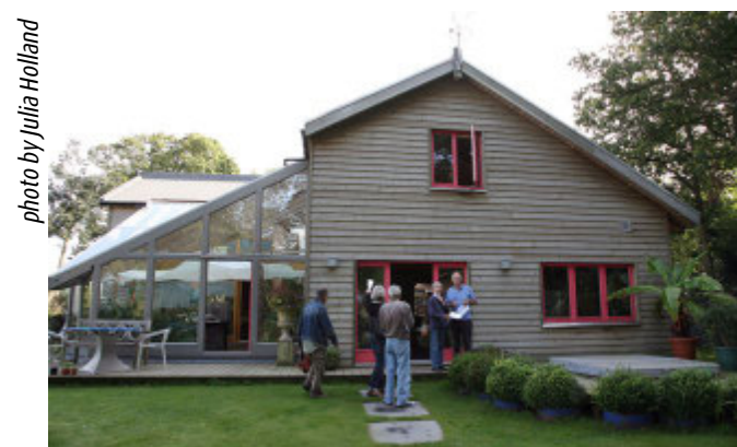
"Ralph's", one of the twelve energy-efficient properties open to the public during CPRE Norfolk's guided tour of "green buildings"
