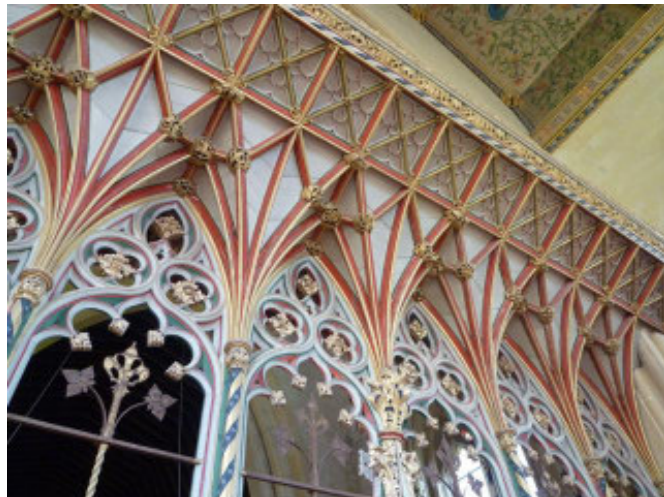
Detail of the Pugin interior of St Mary’s Church
