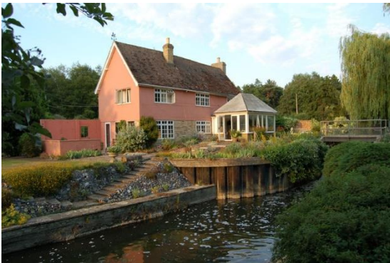
Fullers Mill house and mill stream
